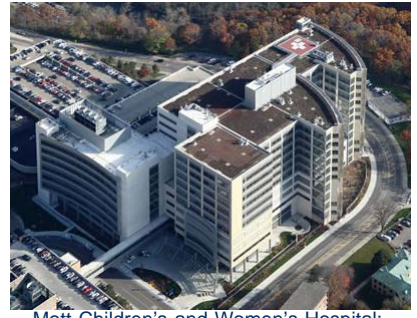
Mott Children's and Women's Hospital: Goal of LEED-NC Certification
