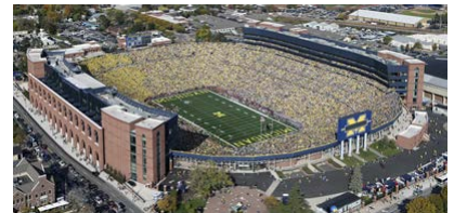
Michigan Stadium Renovation and Addition
